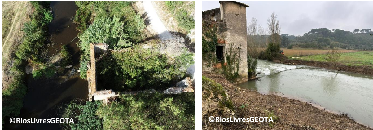
Figure 49. The Vaqueiros weir (at different stages of the project) in Alviela River. For more information visit GEOTA RiosLivres Programme (2023a) .
