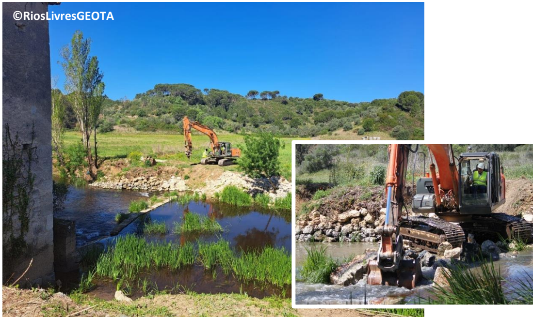
Figure 50. The removal of the Vaqueiros weir required the temporary use of heavy machinery within the channel, which was unavoidable in this case due to the river width. For more information, including video, visit GEOTA RiosLivres Programme (2023a) .
