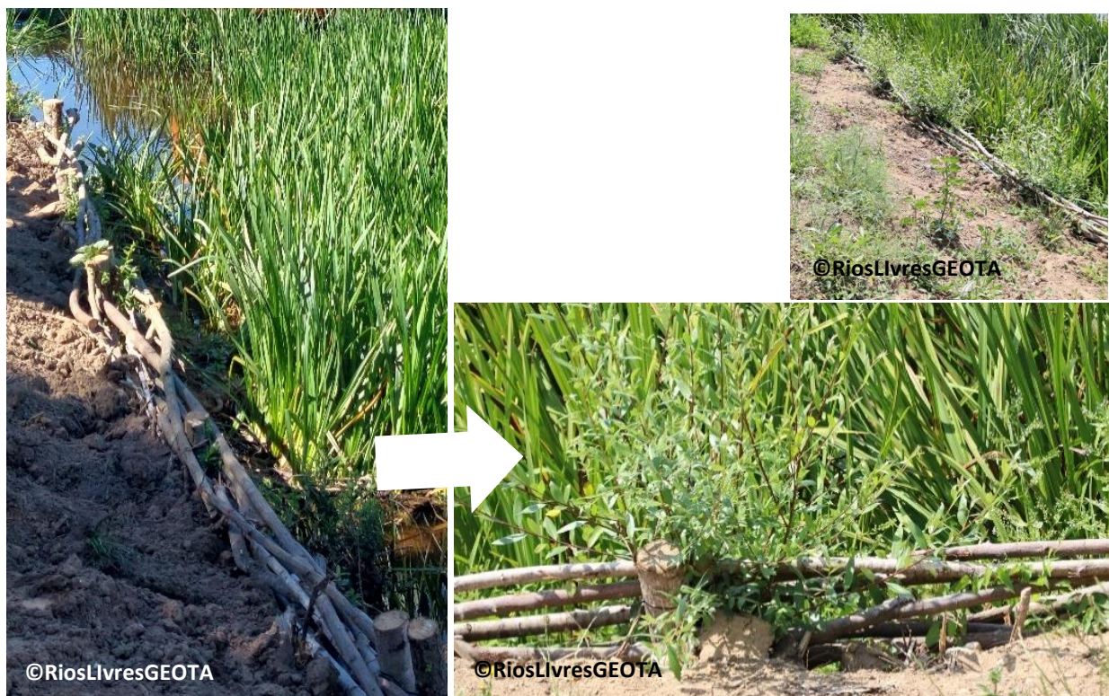
Figure 26. Live willow (native) weaving installed along the stream margin to stabilise the bank and reduce (GEOTA RiosLivres Programme, 2023a).
