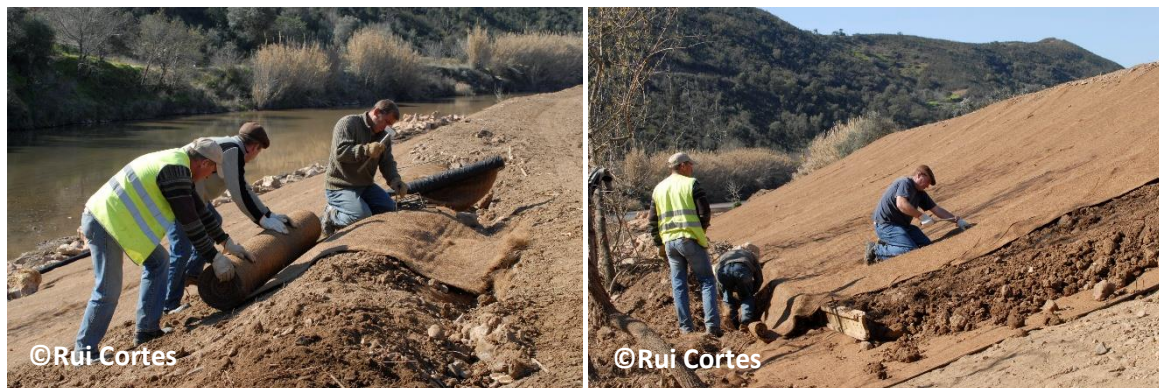
Figure 33. Installation of erosion control blankets, Odelouca River (Tributary of the Arade River, Algarve, southern Portugal), providing temporary surface protection on exposed soils, reducing runoff and sediment loss, and supporting vegetation establishment for long-term slope stabilization. The Odelouca River was characterised by dense and locally riparian vegetation dominated by Narrow-leaved ash ( Fraxinus angustifolia ), willows ( Salix spp.), poplars ( Populus spp.) and alder ( Alnus spp.), with Tamarix and oleander ( Nerium oleander ) occurring in the lower reaches. Large portions of the riparian corridor were lost following the construction of the Odelouca Dam. To compensate for habitat loss, restoration actions were implemented along approximately 180 ha of the left bank, aiming to enhance riparian habitats and support conservation efforts for flagship species such as the endangered Iberian lynx and Bonelli's eagle, including the establishment of the Iberian Lynx National Captive Breeding Centre. ©Rui Cortes
