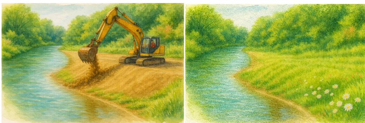
Figure 22. Regrading riverbanks to gentle slopes stabilizes eroding riverbanks, reduces sediment loss, and promotes the establishment of native vegetation, enhancing both ecological habitat and long-term bank resilience. These images illustrate the before and after.
