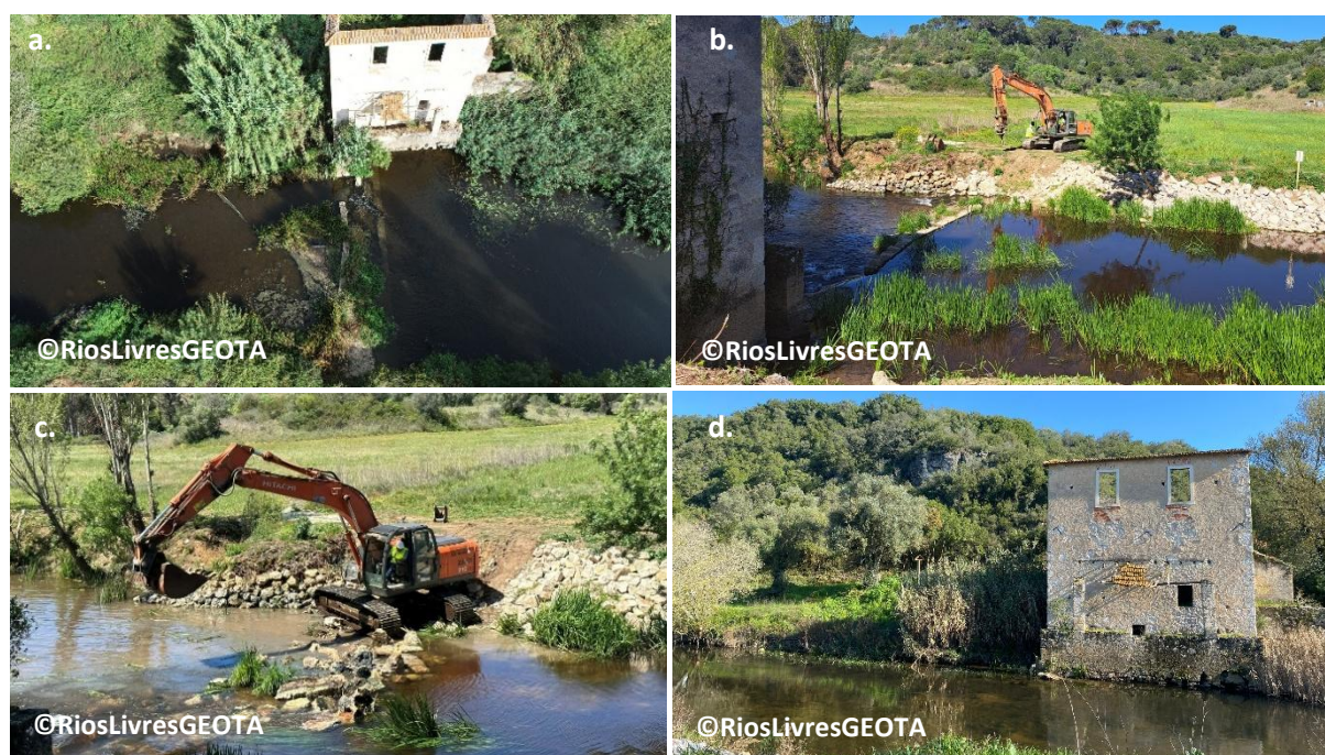
Figure 6. From a. to d. the delicate process of removing an obsolete barrier, a dam in the Alviela River, Tagus Basin Portugal (GEOTA RiosLivres Programme, 2023a). Another example can be found in Mouchlianitis (2024).
