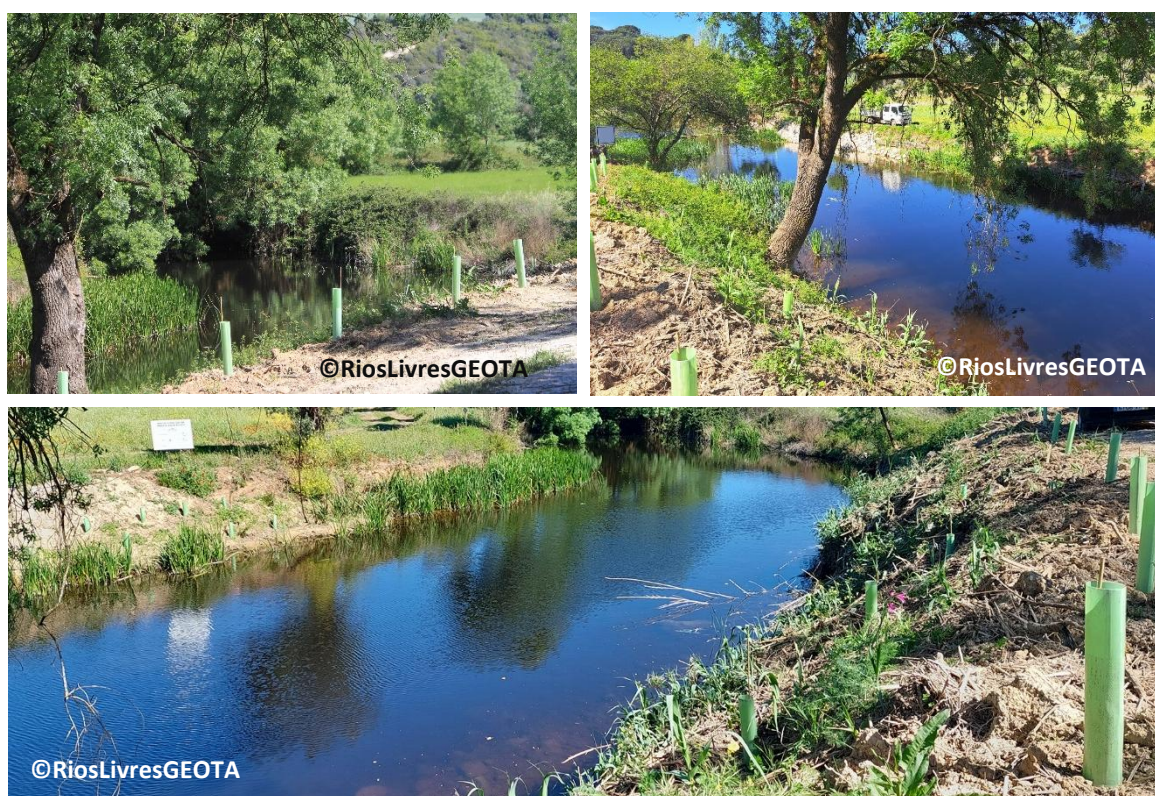
Figure 23. Live planting for riparian corridor streambank restoration, all these images were captured in several phases of rehabilitation of Alviela river at Vaqueiros site, Tagus basin in Portugal (GEOTA RiosLivres Programme, 2023a). See also other projects Friends of the Rappahannock and Hargreaves (2021) .
