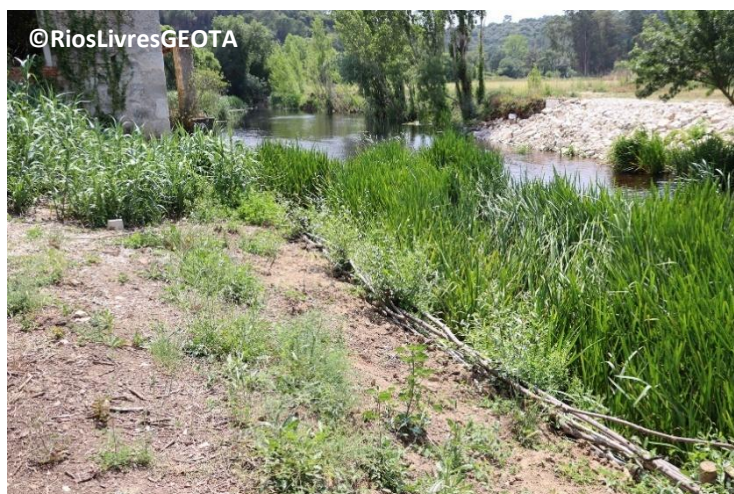
Figure 52. Bank stabilization using live willow (native) fences with woven branches (wood weaving technique) (GEOTA RiosLivres Programme, 2023a).
